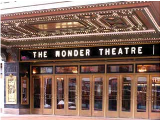
Replicas of the original blade sign (on cover) as well as Wonder Theatre sign and brass doors were installed in 2004.
