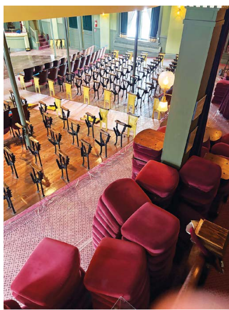
The removal of the existing seats took two days and was done very methodically. First, the seat bottoms and backs are removed and stacked in piles, leaving the stands like soldiers in a row awaiting removal.
