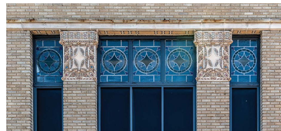
Built in 1921, The Liberty Seneca building originally operated as a financial institution until 2006. Recognizing its charm and cultural potential, South Buffalo native and property developer Jake Schneider purchased the property. With its art deco jewel-box design, stained glass windows, terrazzo flooring, and intact bank vaults, The Caz seamlessly blends historic elegance with modern amenities.
