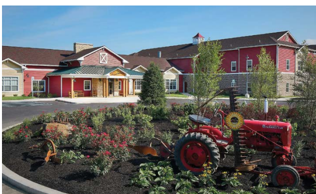
The Olean Manor project is a $10-million-dollar project centering around senior housing in Allegheny. Once complete, Olean Manor will offer senior cottages in an active senior community, located near their assisted living and adult care facility. These new build cottages are scattered on their 40-acre site and offer the community a realistic option for senior members of the community.
