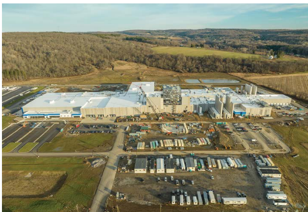
One of their largest investments of nearly $1 billion dollars since its groundbreaking was The Great Lakes Cheese project, brining economic growth and development to the Franklinville/Farmersville area.
