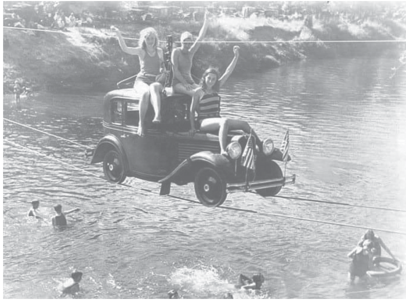
1932 American Bantam Converted for use as a cable car to cross the Pudding River in Oregon. The operator removed the tires and attached 3 cables for stability. It was said 1 gal of gas was good for 1500 trips across the 120 ft span.
