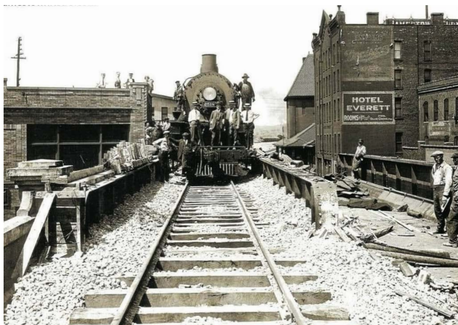
1st Train to Cross the Main St. Railroad Bridge. June 2, 1925 • Jamestown, NY
