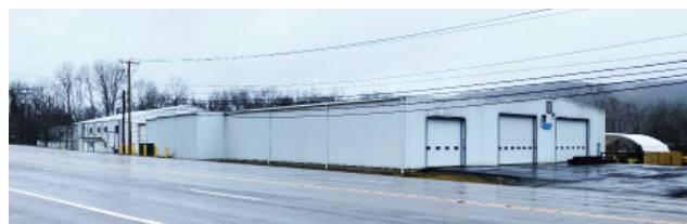
45,000 square foot former Sanzo Beverage Distribution Center on Route 16 in Hinsdale, NY. The Cattaraugus County IDA was instrumental in assuring they secured this new location.
