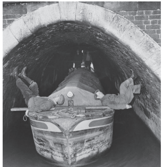
Legging was the method of getting a boat through a tunnel. On short tunnels, the legging was done by the boat, owner and crew. At Long tunnels, professional leggers were available.
