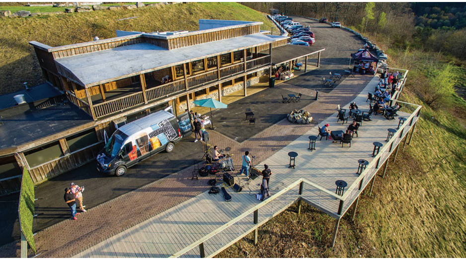
Apollo Canna Co. is located at 380 Parkway Drive in Salamanca, NY, formerly the Red Garter Restaurant.
