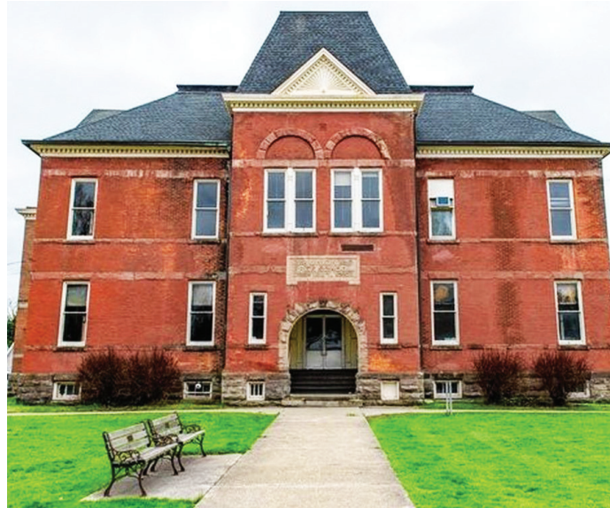
The Village Board of Ellicottville will apply the 1887 Building NY into the Forward and Restore NY program which offers economic assistance initiatives to encourage community development.
